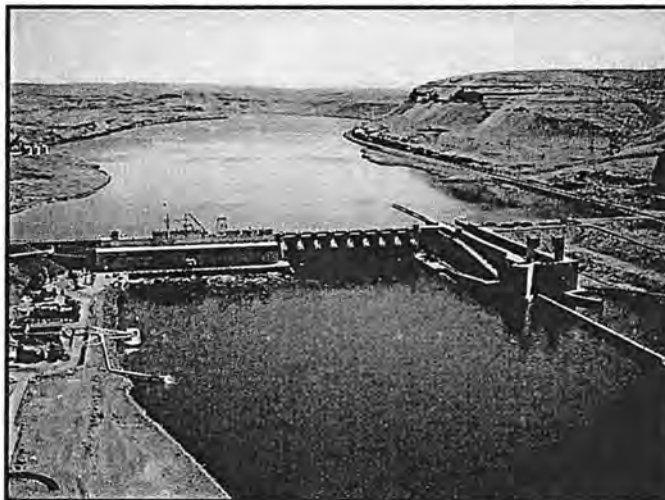
Lower Monumental Lock and Dam on the Lower Snake River. Photo source: U.S. Army Corps of Engineers
