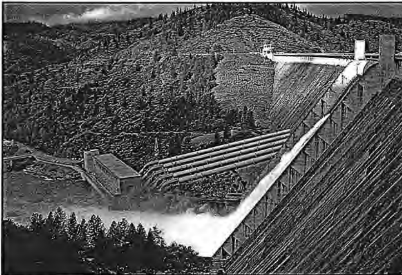
Shasta Dam (CALIFORNIA). Photo Courtesy of U.S. Bureau of Reclamation
