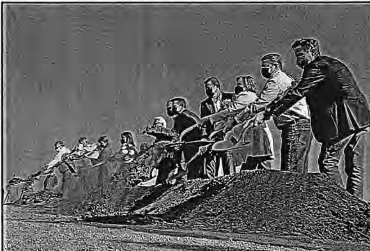
The Bureau of Reclamation, Friant Water Authority, and California Department of Water Resources last January celebrate the groundbreaking of a $187 million construction project to restore capacity in a 10-mile portion of the Friant-Kern Canal.
