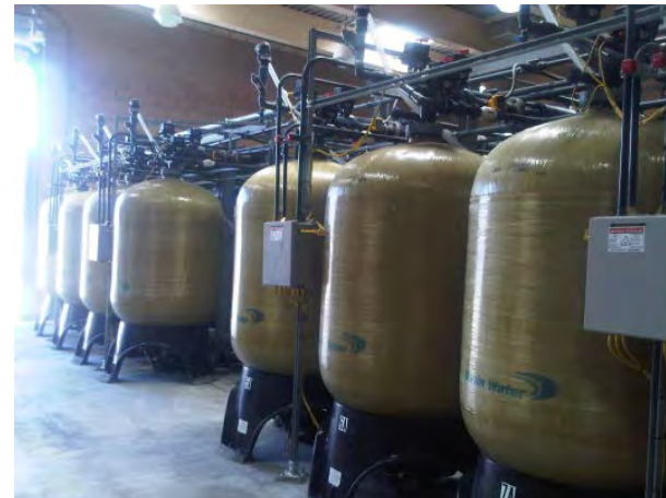
Strong-Base Anion Exchange with Residuals Treatment (SBA)
